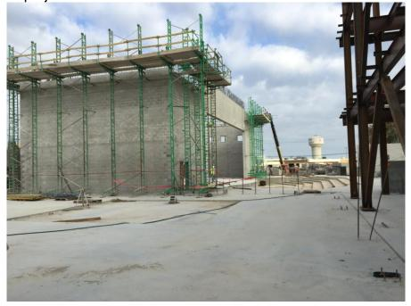
**PERFORMING ARTS CENTER** (PAC) – Block walls are being erected at the PAC stage, the stage fly loft and back of stage.
