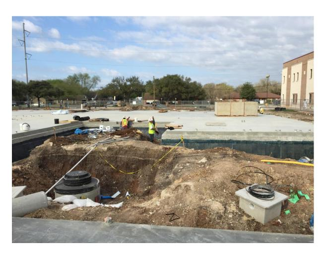
CAREER TECHNOLOGY CLASSROOMS - The concrete foundation has been poured at the Veterinary Classroom and Lab. Concrete earth retainers, waterproofing and backfill are in progress.
