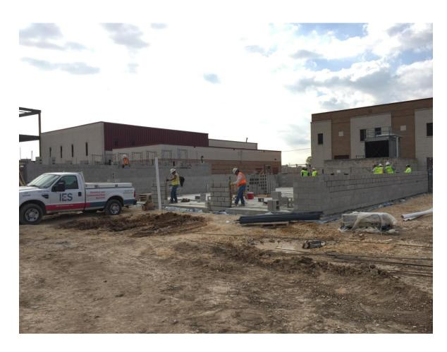
**CHILLER BUILDING** – Concrete walls being erected. This building which is located north of the Freshman Center will house the mechanical equipment for the school.
