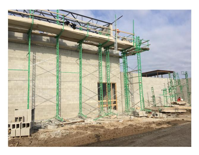
**GYMNASIUM** – Concrete block walls are being erected at the east wall of the secondary gym. The east wall of the gym faces the current weight room and the stadium.
